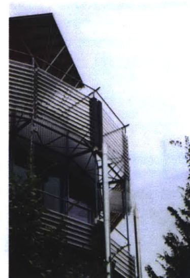
evacuated tube collectors
