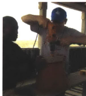
Drilling the 1" hole
