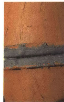
Figure 47 SBR Bond Used to Seal Two PHW CPFs
