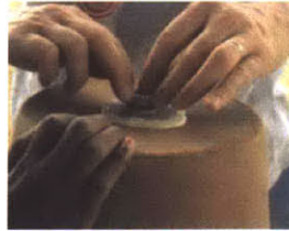
Pushing another O-ring onto the top of the PVC riser pipe
