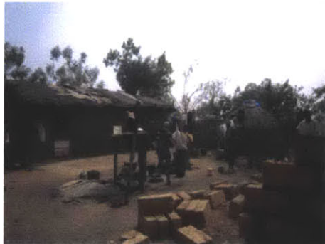
Houses in Compound (Forefront Structure is House in Construction)
