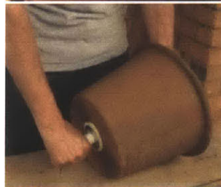
Removing the PVC pipe by first twisting it free and then pulling it out
