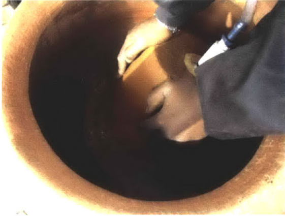
Figure 43 Leak Testing the Completed KWK
