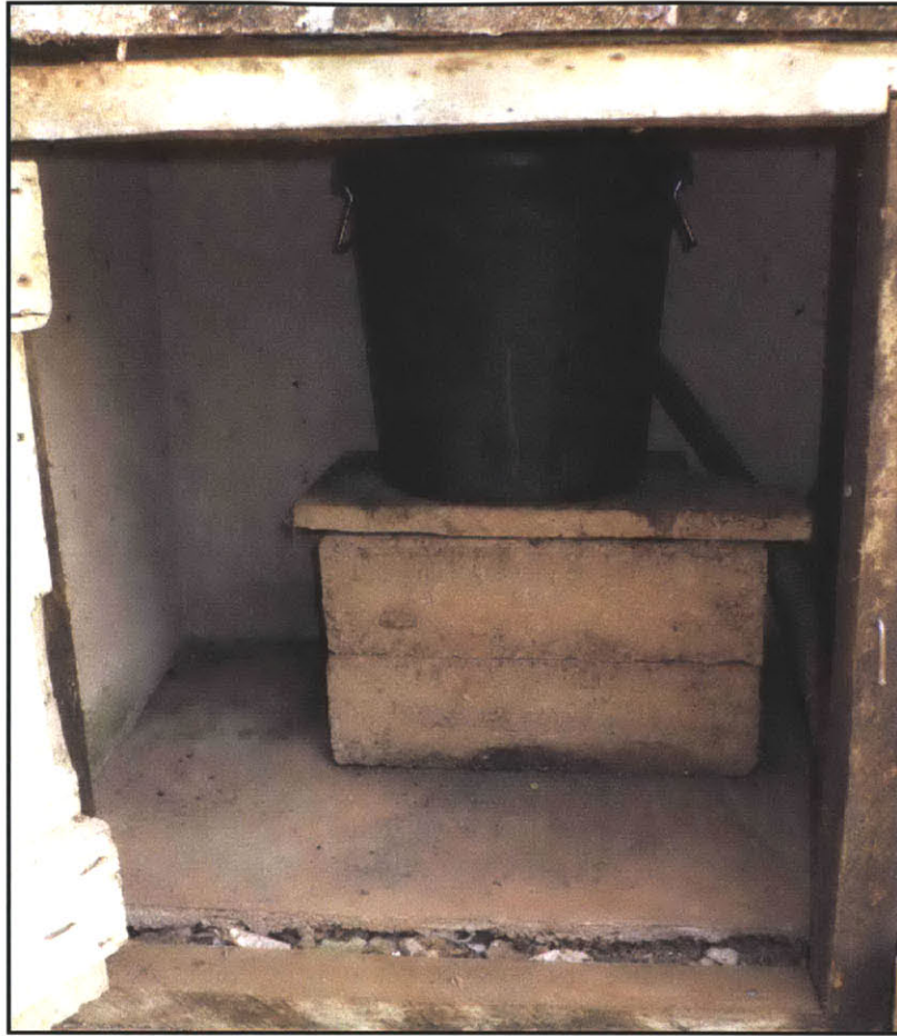
Figure 5-8 Removal Bucket at the back of the EcoSan latrine and urine diverting pipe
