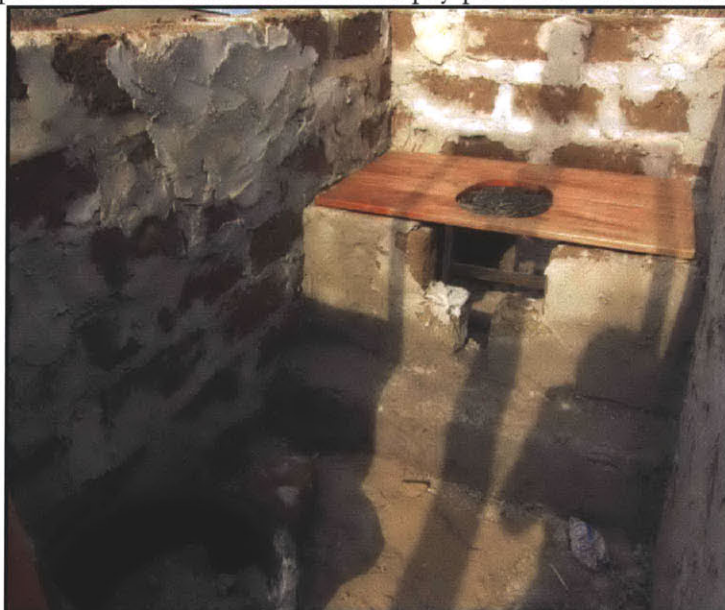
Figure 7-4 Interior of latrine structure in mid-construction (Photo credit: Mette Andersen)
