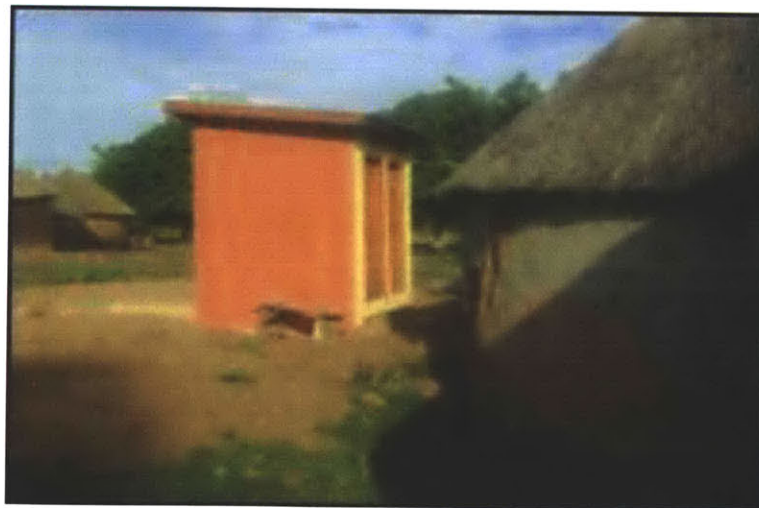
Figure 5-5 Latrine built for the home of Mahamud Sugli in Taha Village (Photo Credit: Ernest Akkakia)
