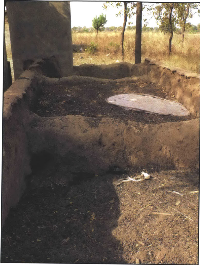
Figure 5-7 Three-Compartment Composting Pit next to the EcoSan pilot latrine
