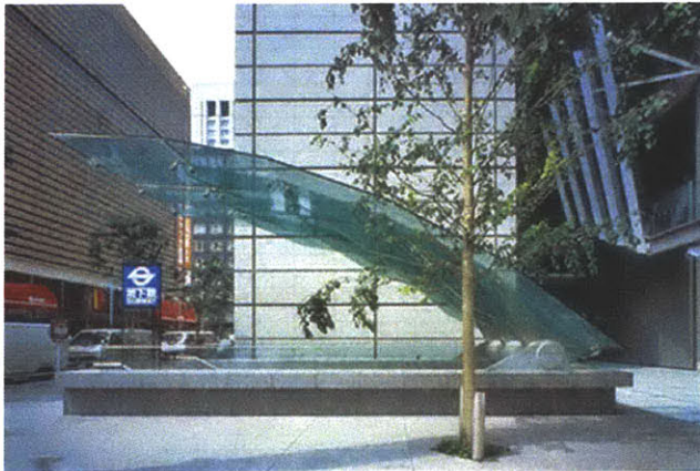
Figure 6. Cantilevered glass canopy in Tokyo, Japan [1].
