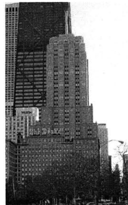
Figure 2.10 Palmolive Building in 1929
