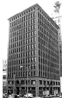
Figure 2.4 Guaranty Building in 1895
