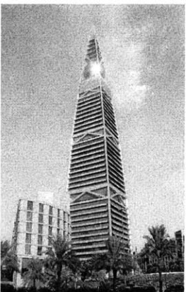
Figure 2.34 Al Faisaliah Center in 2000
