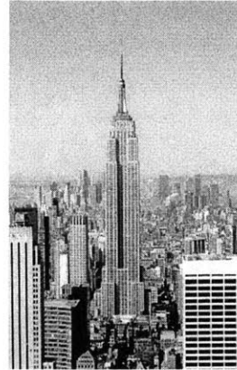
Figure 2.12 Empire State Building in 1931
