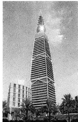
Figure 5.12 Al Faisaliah Center in 2000
