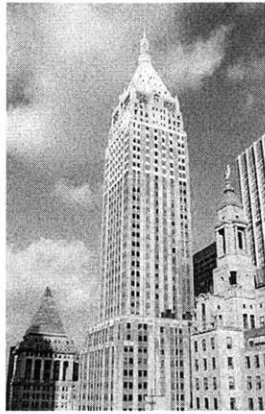
Figure 5.13 40 Wall Street Building in 1930
