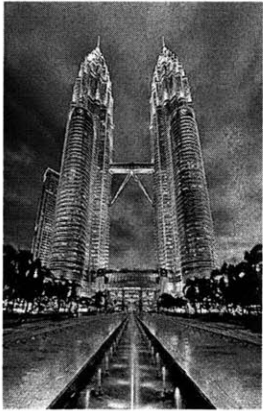
Figure 2.32 Petronas Towers in 1998
