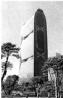
Figure 5.11 Pearl River Tower under cons.
