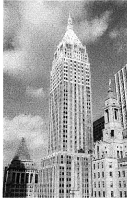
Figure 2.11 40 Wall Street Building in 1930
