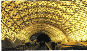
Fig.08-2: paper tube roof structure of Japan Pavilion by Shigeru Ban
