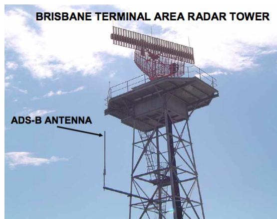
Figure 8: Temporary Installation of an ADS-B Antenna on a Terminal Area RADAR Tower in Brisbane, Australia (credit: Greg Dunstone)
