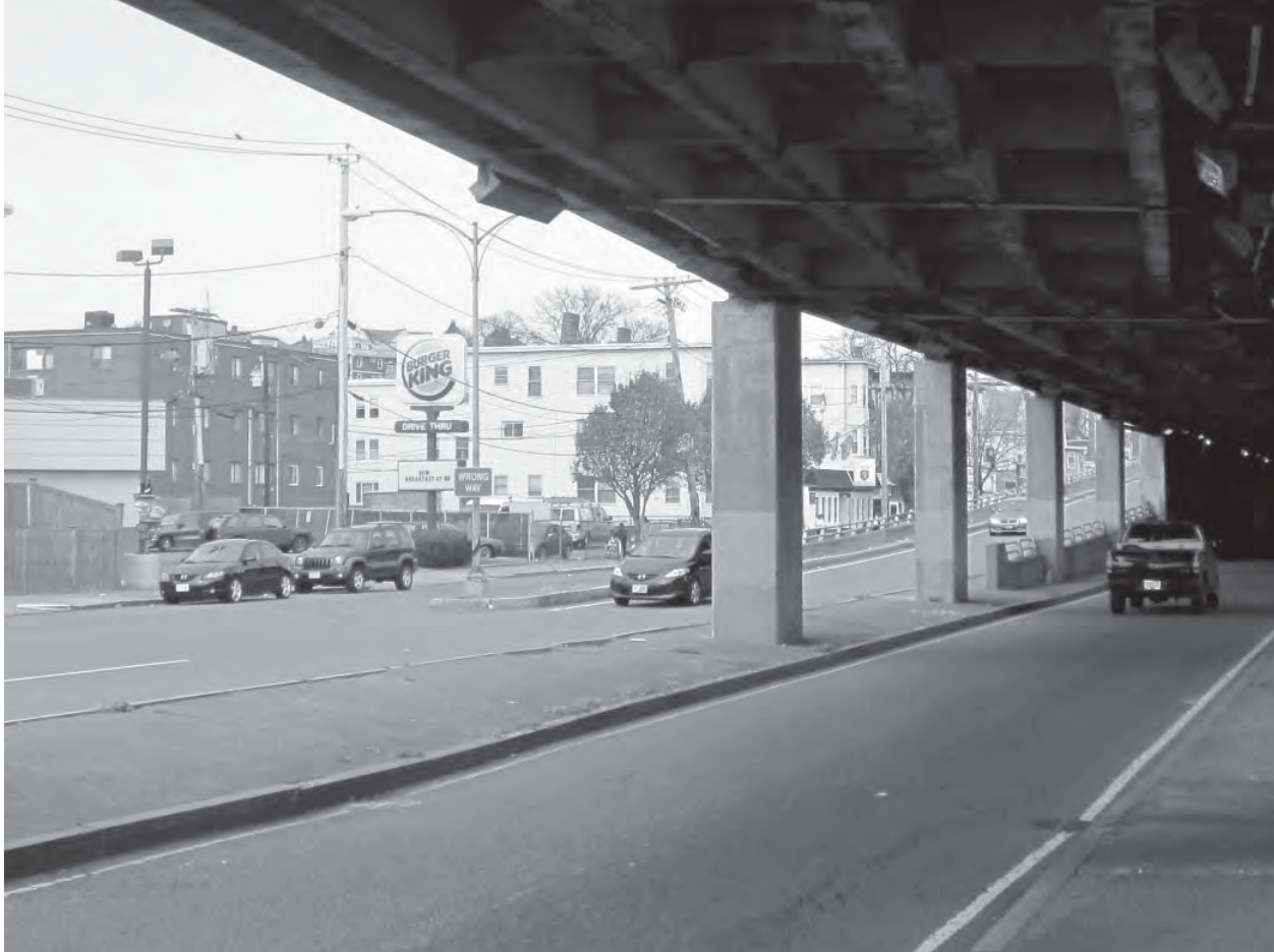
Figure 2: Streetside View of McGrath/O'Brien Highway (near intersection with Washington Street)
