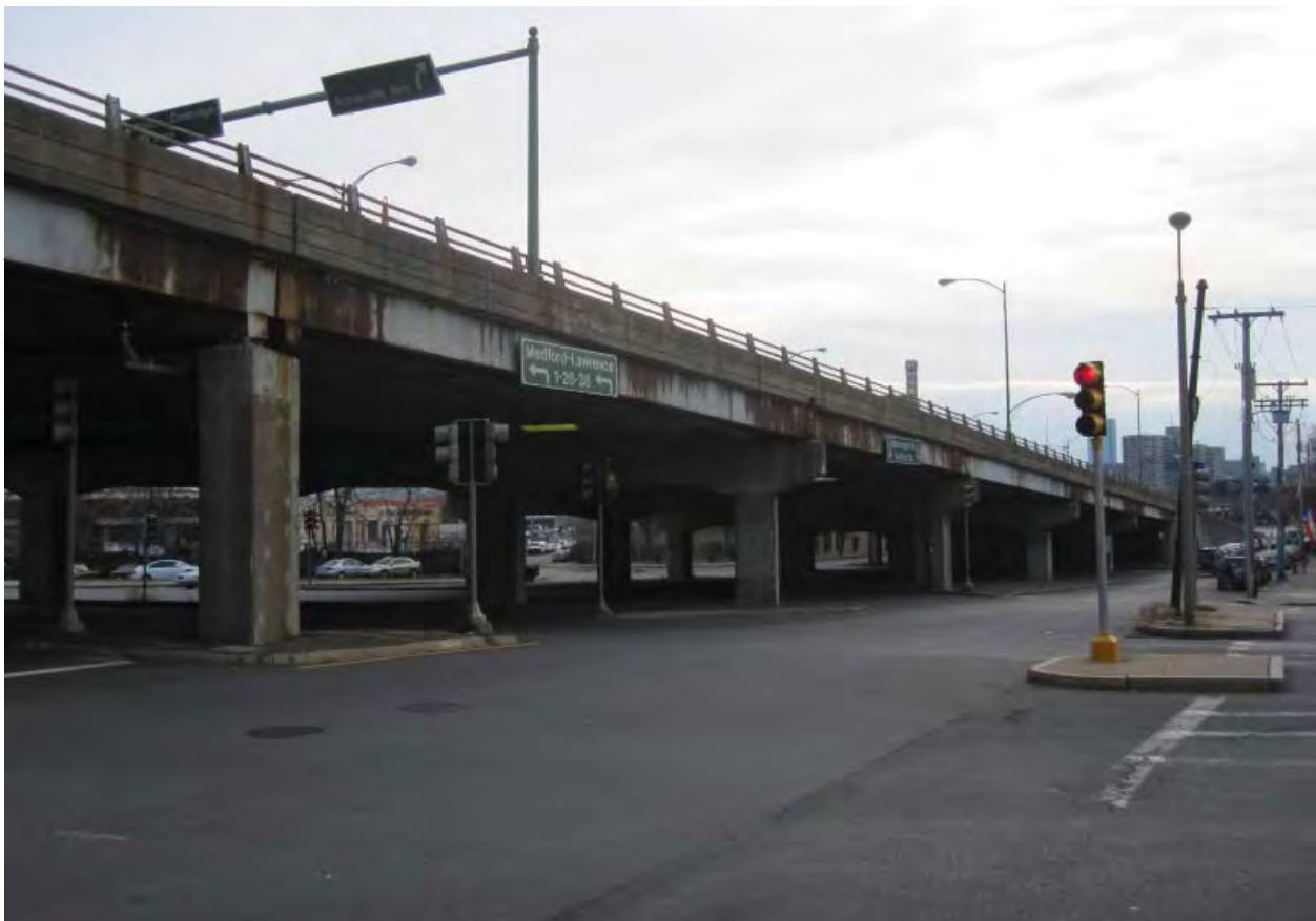
Figure 9: Streetside view of McGrath/O'Brien Highway (intersection with Washington Street)
