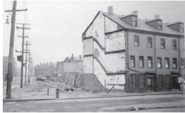
Figure 15: Demolitions along the route, 1925. (Courtesy of Cambridge Historical Commission)
