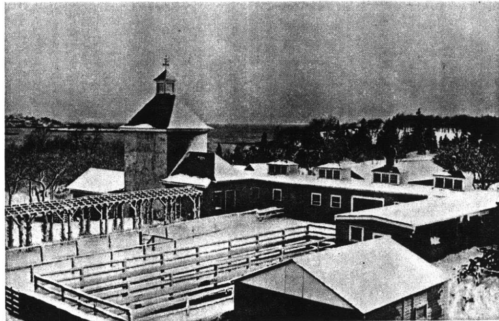
129. Brewer Estate Barn, World's End in background, 1932.
