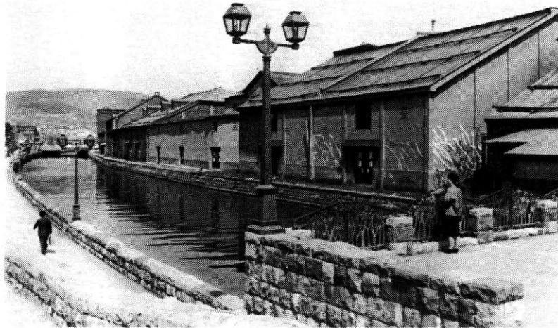
Figure 5-31: Entry and Orientation Area (4)
