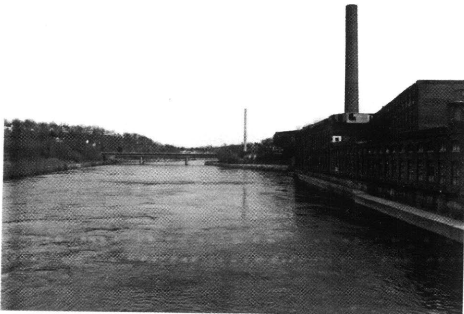
Figure 4-3: Merrimack River and Massachusetts Mill
