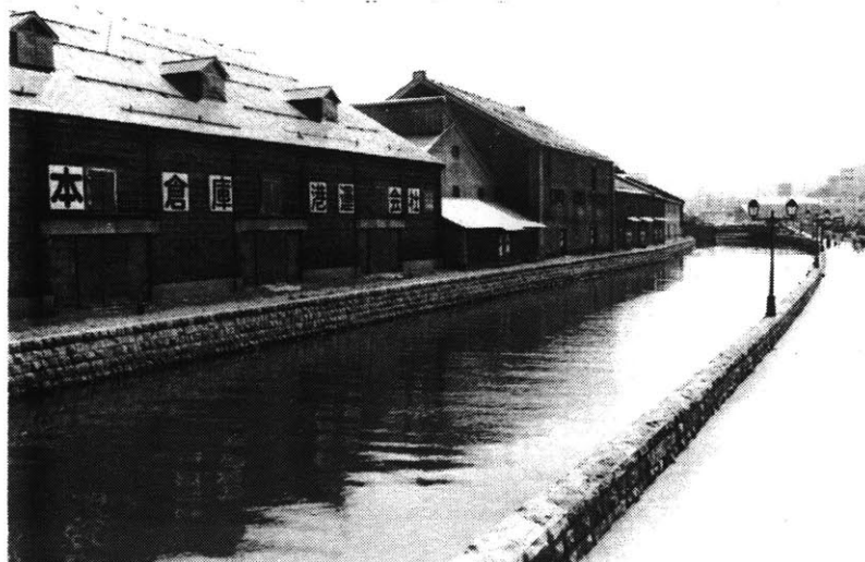
Figure 5-29: Entry and Orientation Area (2)
