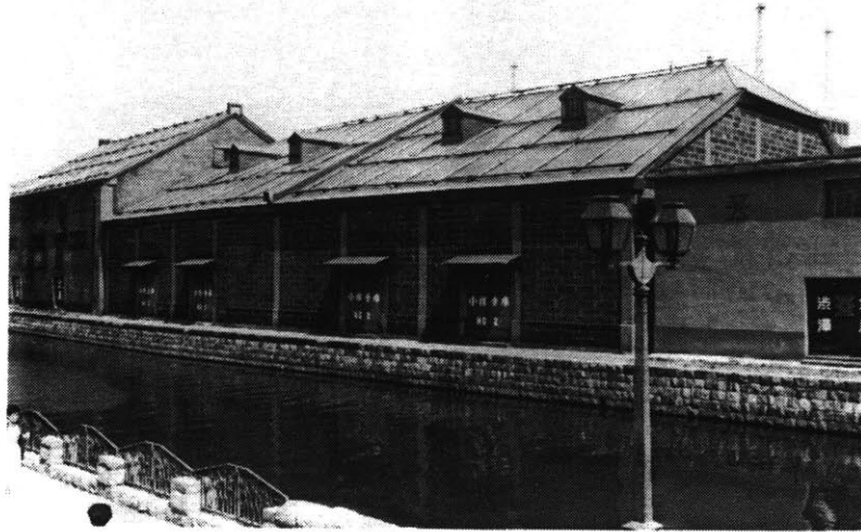
Figure 5-28: Entry and Orientation area (1)
