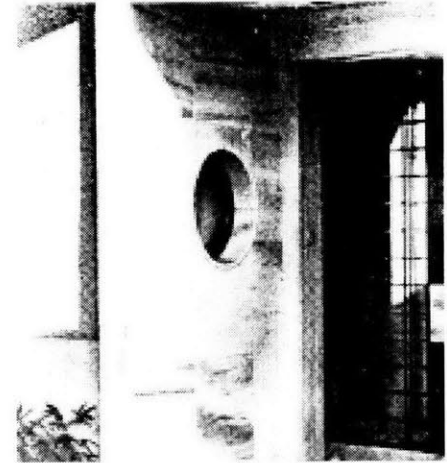
Fig.4.13 Zeki Sayar, Cili Apartment, Main entrance Gumussuyu/Istanbul, 1936
