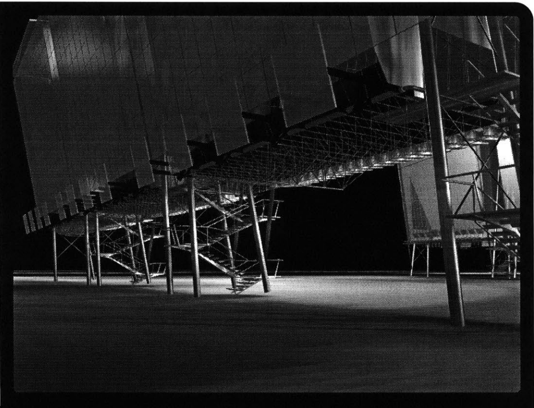
fig. 60: view below looking across and northeast in the Altmarkt
