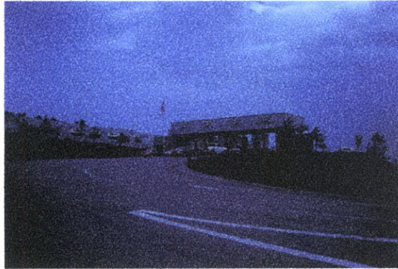
61 Toll booth entry
