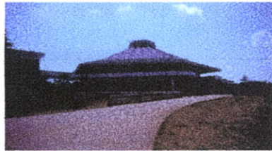
42 Approach from parking lot
