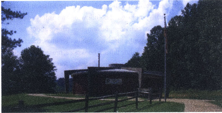
32 Approach from parking lot.
