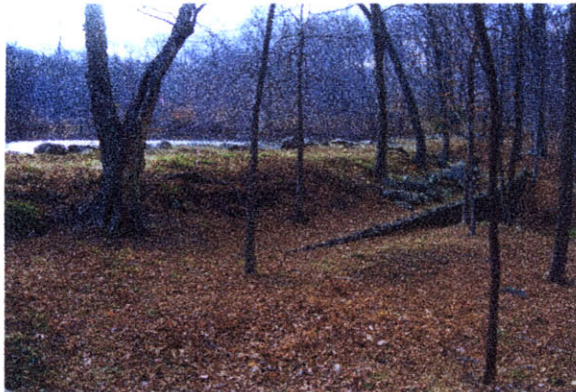
23 Concrete wall in the woods
