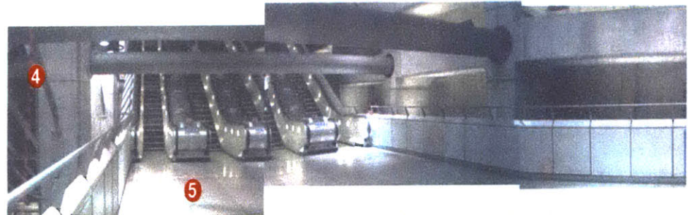
Inside the circulation collector volume of Westminster Station
