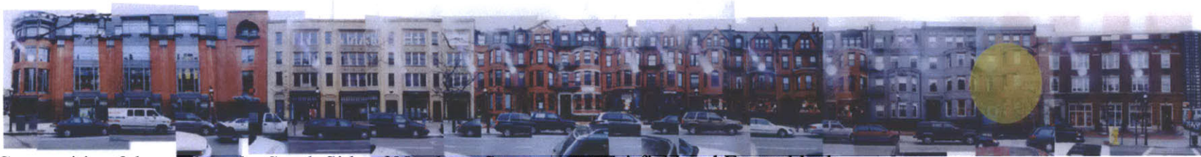
Composition 2 located on the South Side of Newbury Street on the Fairfield and Exeter block. The in-fill site is highlighted.
