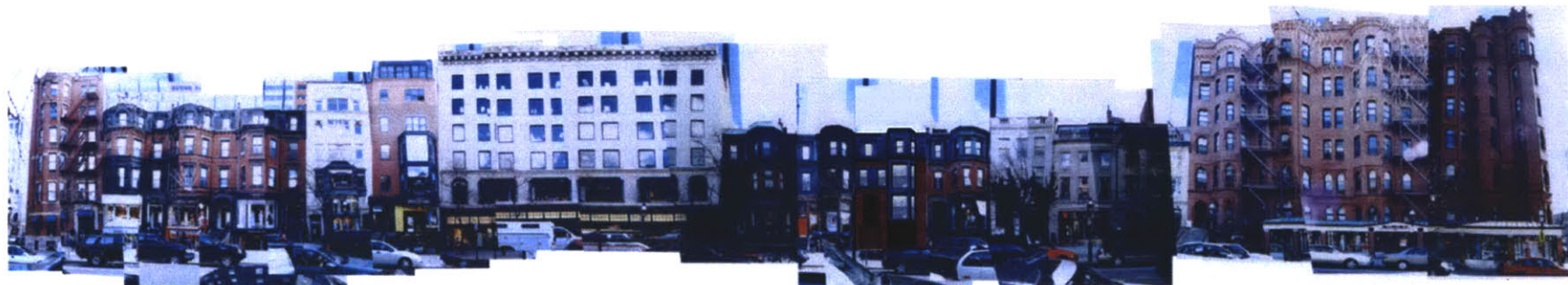
Facade within the existing context
