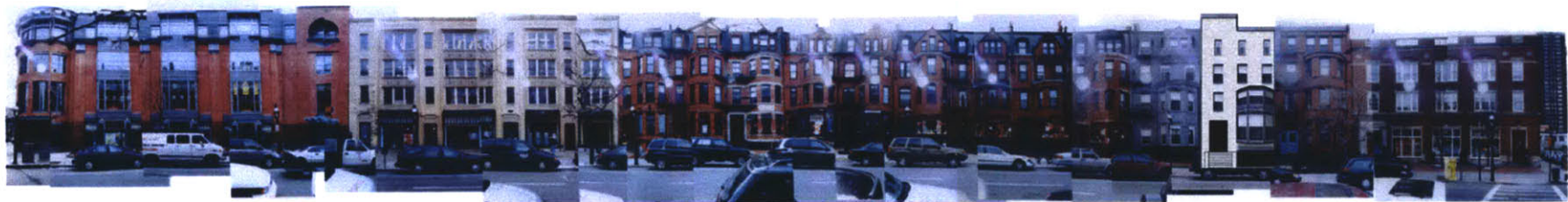
Facade within the existing context
