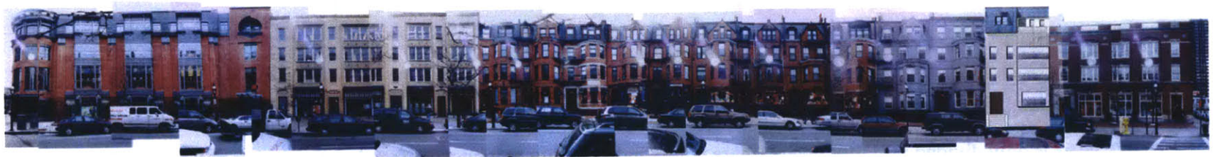
Facade within the existing context
