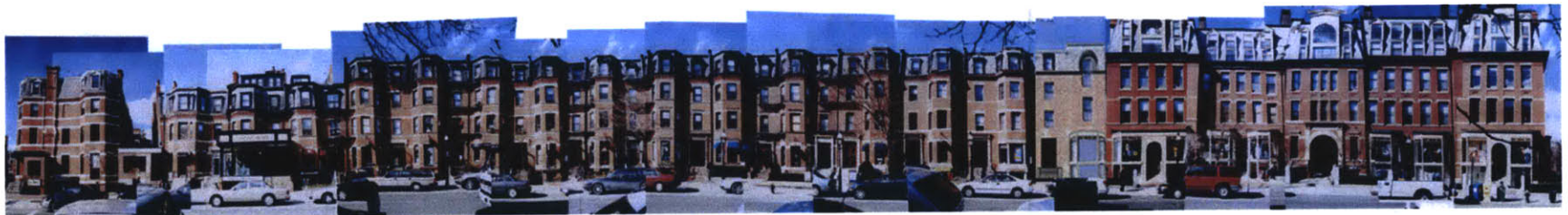
Facade within the existing context
