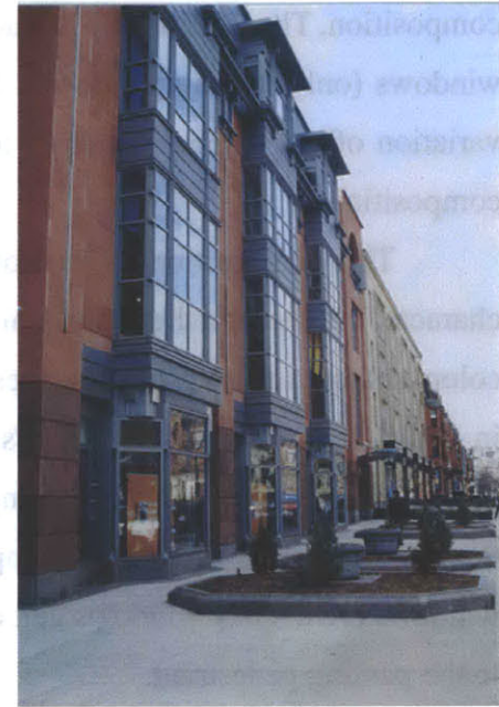
Photograph 2. The relationship between the bay windows of the first floor
