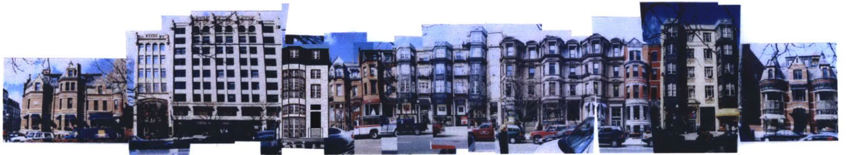
Facade within the existing context
