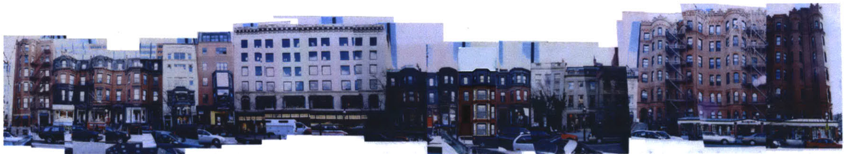
Facade within the existing context
