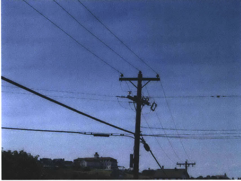
Figure 3.4: Three-Phase Powerline Configuration
