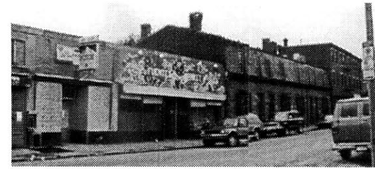
Figure 38: Existing mixed-use buildings along Parker Street
