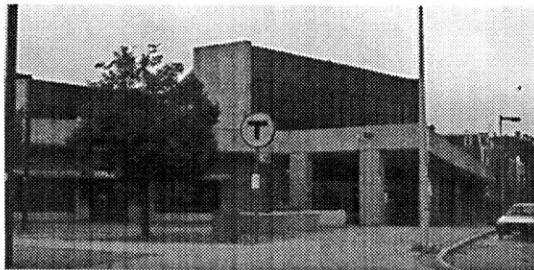
Figure 29: The new Roxbury Crossing MBTA Station
