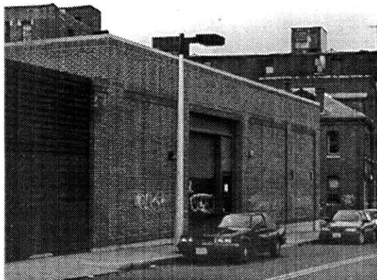
Figure 65: Existing MBTA power substation
