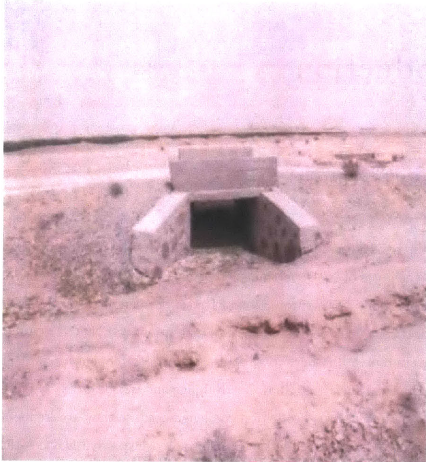
Figure 1-1: A culvert typical of those for which routine investigation is required.
