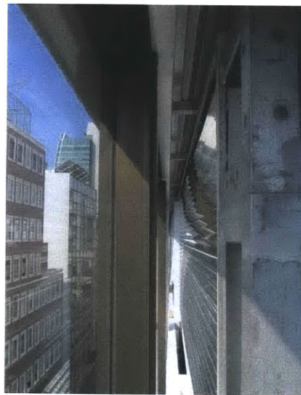
Figure 6.19: View of the Shading Caused by the Building Overhang
