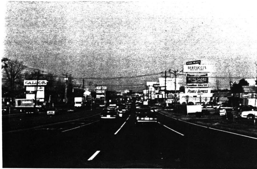
The expanse of Route 9 features road, signs, cars and low-lying stores of every shape and style.
