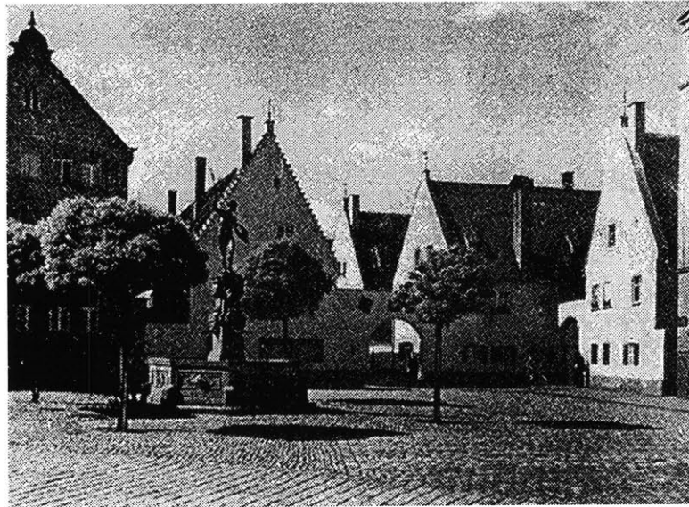
Figure 14. The first known social housing project on German soil— The Fuggerei in Augsburg, 1519 64
