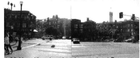
1.28 New Housing developments at Brannan St. along the Embarcadero
