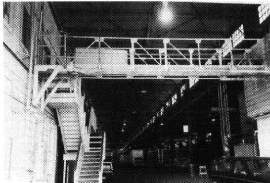
1.69 Interior view of Pier 28's metal structure.
