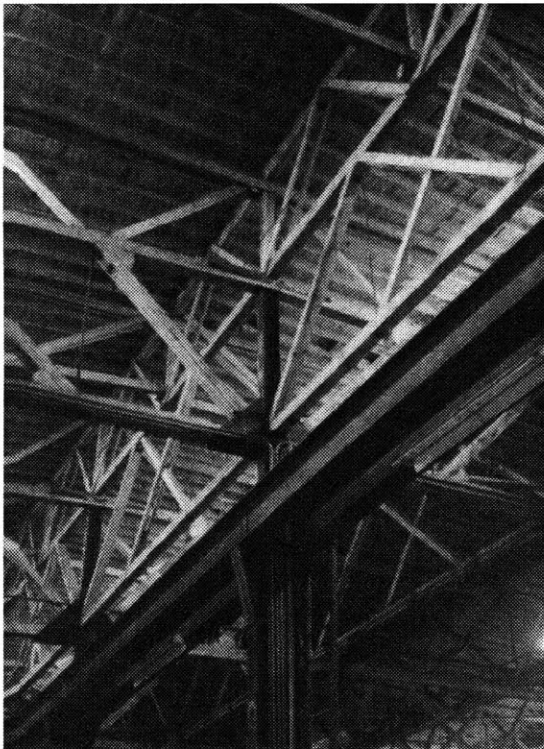
1.59 Looking up under a central column
