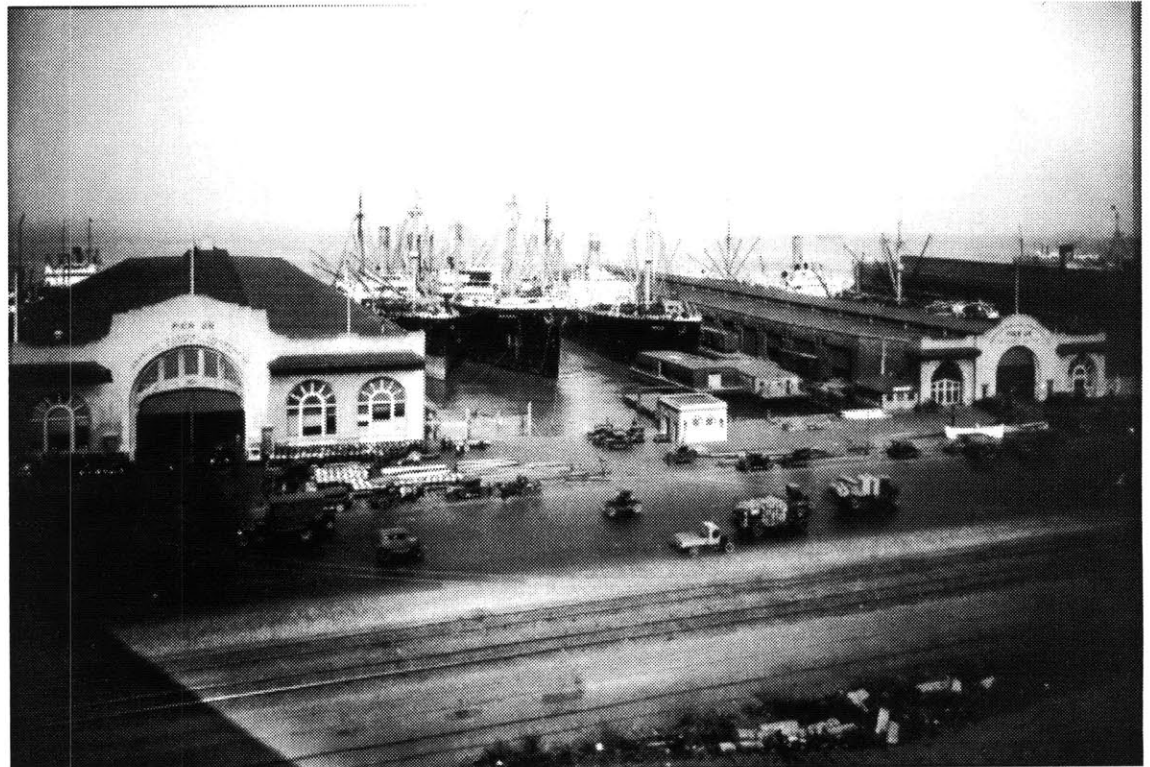
1.36a View of Pier 26 and Pier 28, 1915.
