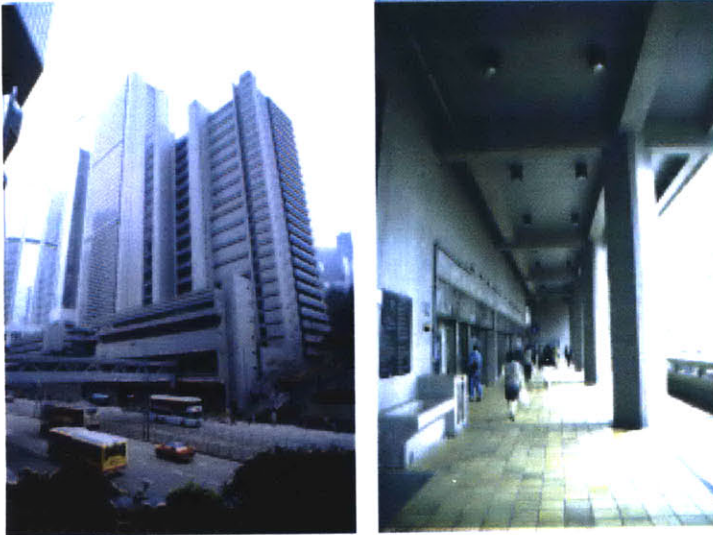
fig. 6.19 & 6.20 Photographs showing the upper level pedestrian footbridge connecting individual's tower podium structures.
