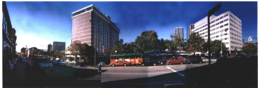
Fig 5.1 View from Cambridge Street to Charles River Plaza (site)
