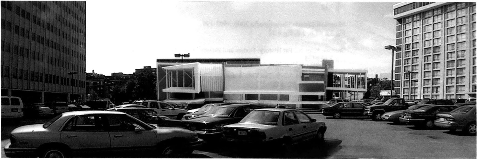
Fig 8.18 view from the upper mezzanine parking lot
