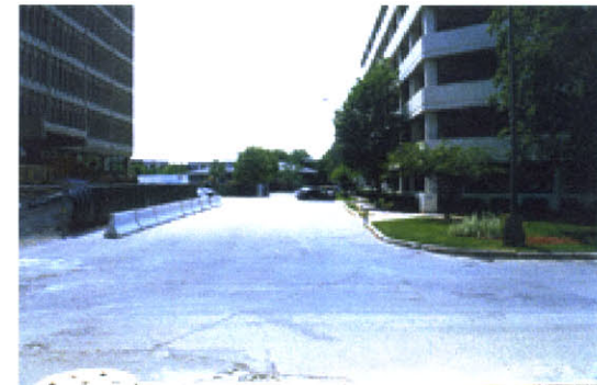
view of the site facing east
