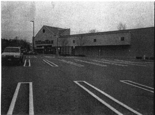
OfficeMax (note the peaked roof).
