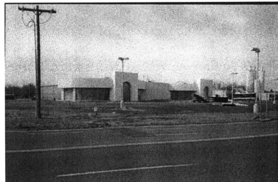
New sprawl construction.
