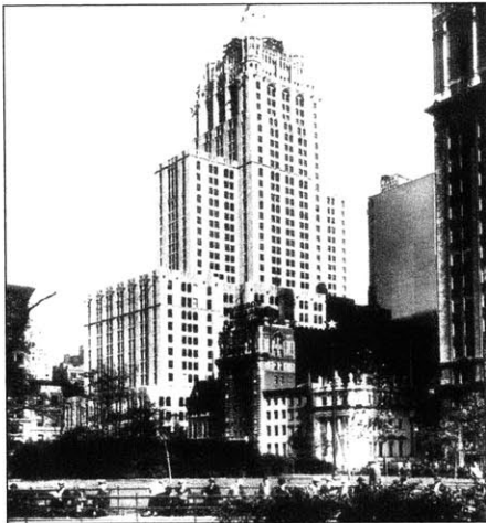
Figure 1.8 The New York Life Insurance Building, one of the first buildings to be designed with noise insulation as a goal. Source: The Soundscape of Modernity
