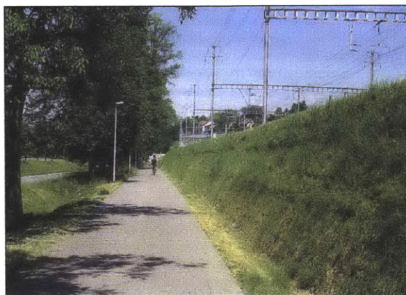
Figure 3.7 A photograph of a structurally reinforced bio-barrier separating the rail line from a walking path. Source: Environmental Noise Barriers
