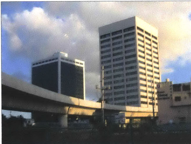
Figure 5.18 View of Tren Urbano guideway and office towers near Roosevelt Station. Source: Author
