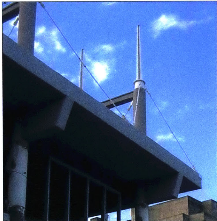
Figure 6.1 The tensile supports at Pinero Station evoke a modern feel. Source: Author
