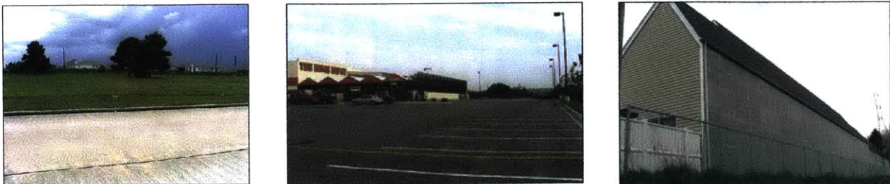
Figure 3.9 The U.S. Department of Transportation’s published examples of “Noise Compatible Land Use Planning.” From right: open space buffering residential uses, retail setback from highway with large parking lot, the blank wall of a townhouse. Source: Entering the Quiet Zone: Noise Compatible Land Use Planning .
