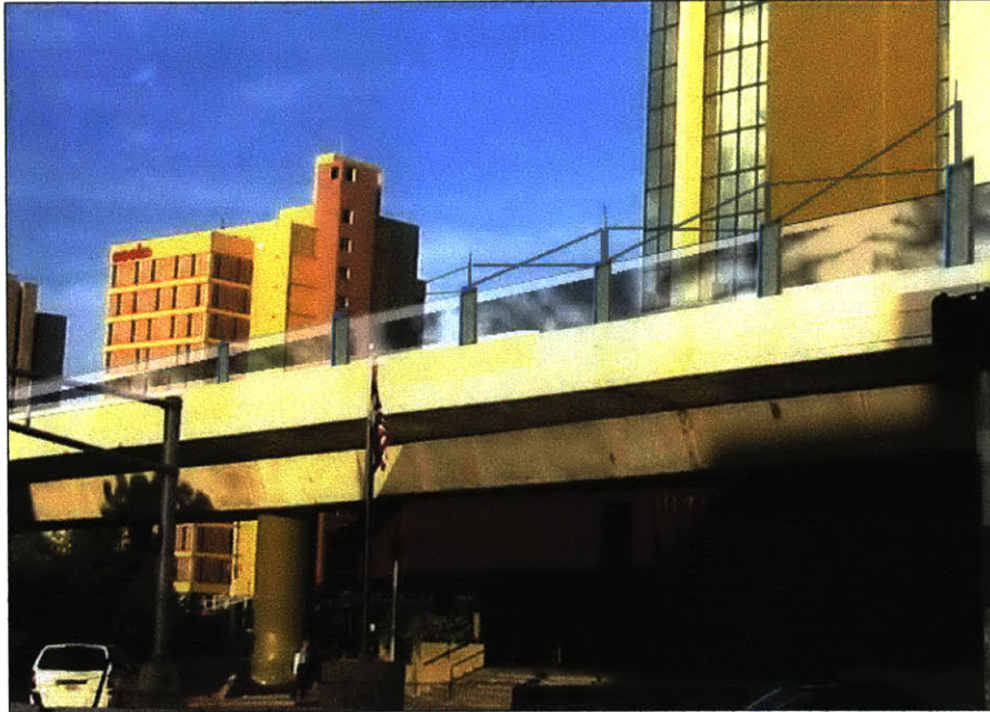
Figure 6.2 Superimposed image of Tren Urbano guideway near Domenech Station with additional noise barrier constructed on existing guideway. The glass noise barrier has tensile supports, mimicking the architecture of Pinero Station.
