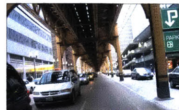
Figure 1.3 Parking structures lining the street adjacent to the El. Source: Author
