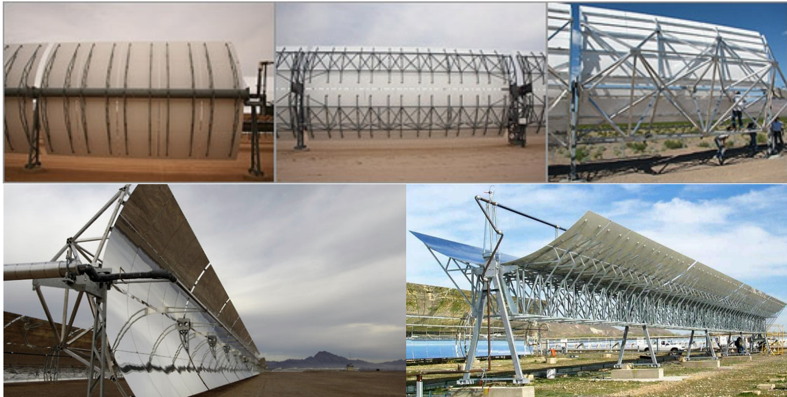
Figure 2-12: Structural designs of existing parabolic troughs [12].
