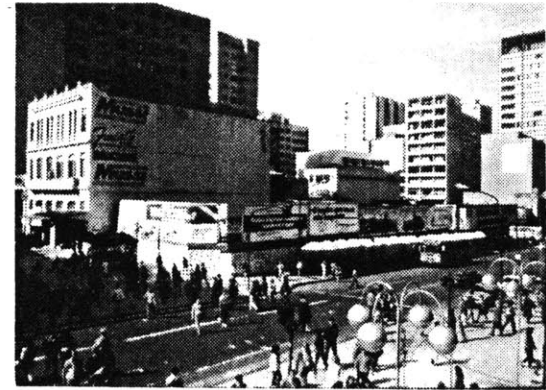
The intersection of Rua das Flores and Rua Marechal Floriano. The building next to the empty lot protrudes 2 meters into the street.
