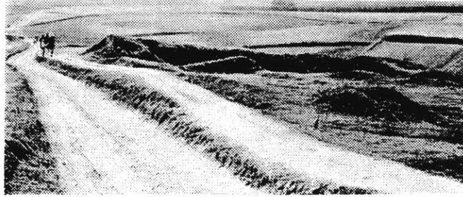
1959, BUILDING SITE OF LSM
