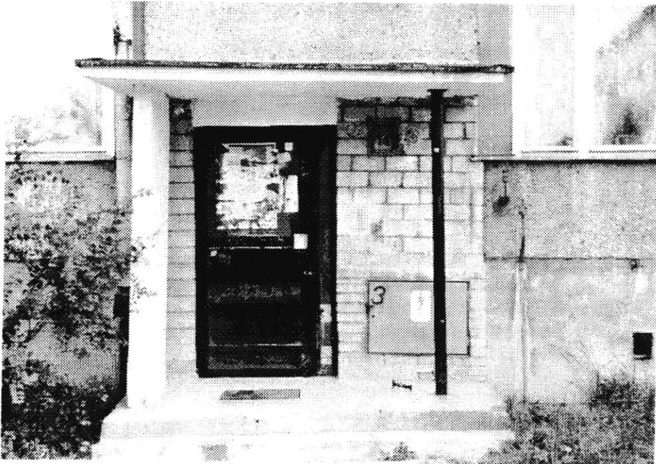
TYPICAL ENTRY DOOR OF HOUSING BLOCKS
