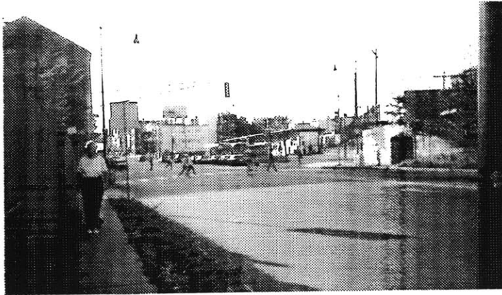
Figure 3-4: Site view from the east - Cambridge Street
