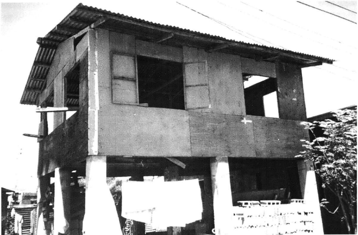
Plate 5. Variations in House Construction: Sagayad (I)
