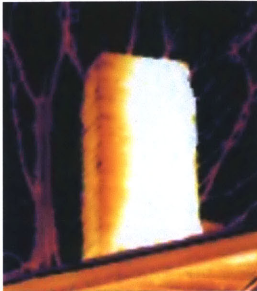
Figure 23: Infrared image of chimney loss
