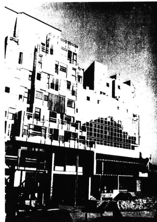
LUCIEN KROLL and ATELIER, Medical Faculty buildings . University of Louvain, Woluwe St. Lambert, near Brussels, 1969-74. An artificial hill town of various activities, articulated with different building systems.
