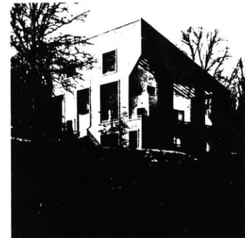
Partial transparency of the lattice porch façade (above)
