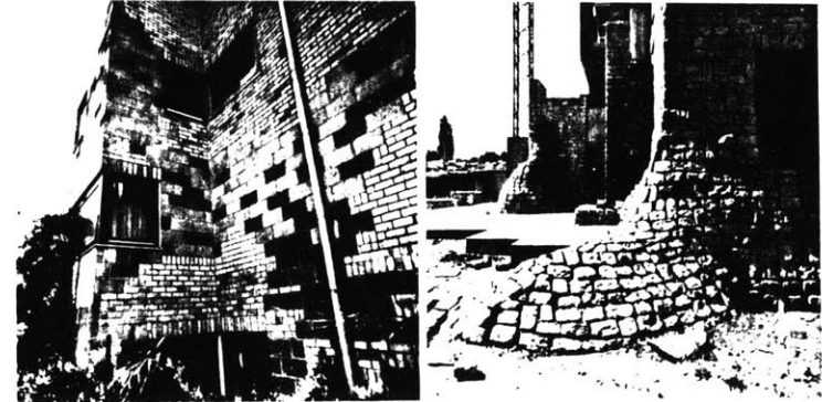
3 One day we said to the builders 'mix with bricks as you see fit; you start here and go at least up to there' 4 We suggested the general form and the builder invented the shapes.
