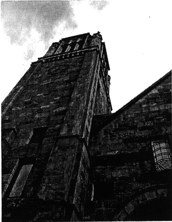
left: Window detail [tower].
