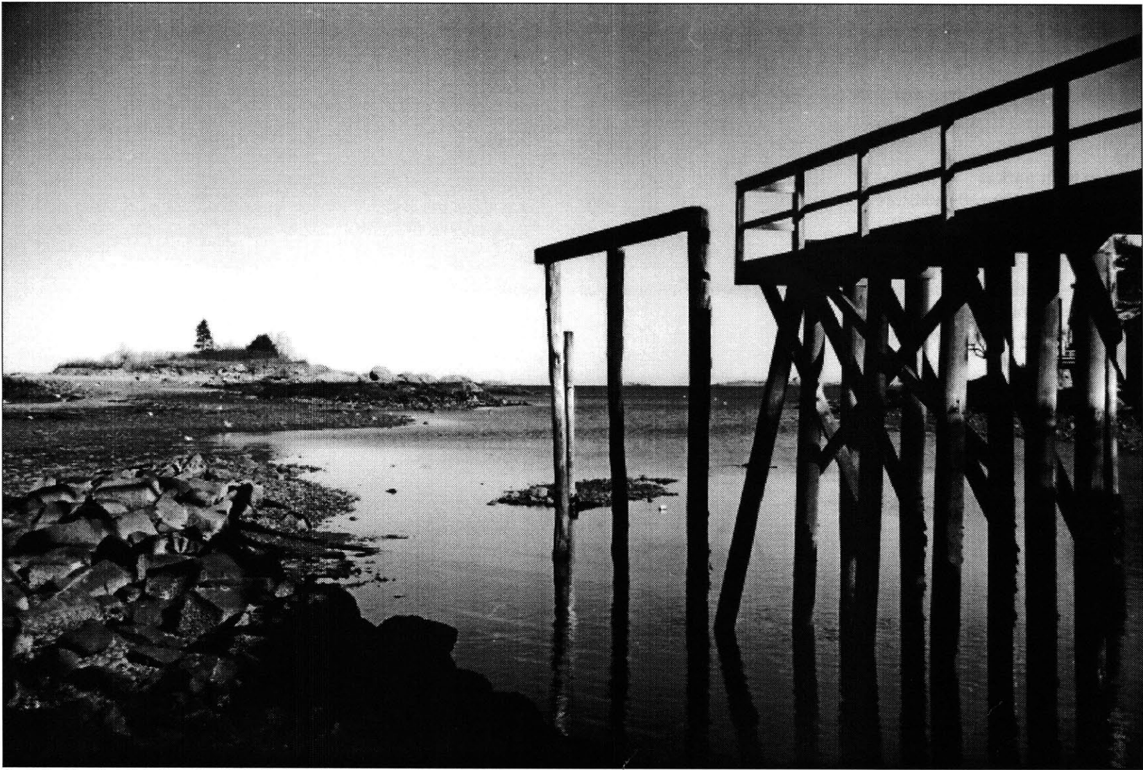
fig. 2.1 Abandoned dock in the Little Harbor, Marblehead, Massachusetts
