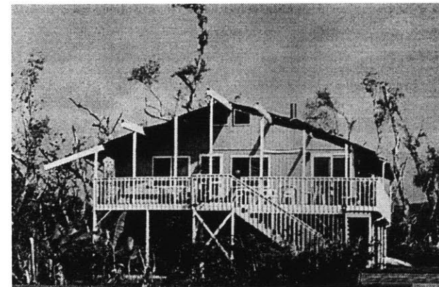
Top: Typical wall connections with hurricane straps (Southern Building Code Congress International 80) Bottom: Excessive roof overhangs and poor connections led to roof loss (United States, Federal Emergency Management Agency 43)
