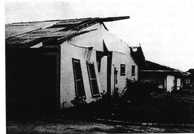
Top: Gable end walls were especially vulnerable at the cripple wall studs (Ronald A. Cook and Mehrdad Soltani 517) Bottom: Gable roof end wall failure (Structural Engineers Association of Hawaii, A Survey of Structural Damage Caused by Hurricane Iniki 30)
