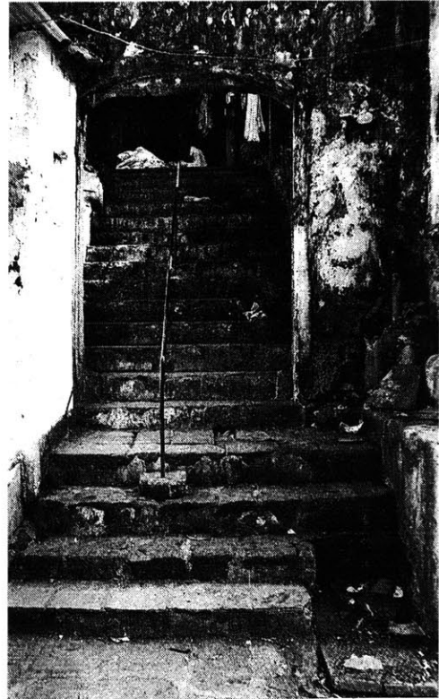
Fig. 28 Steps leading into a private residence from the inner street
