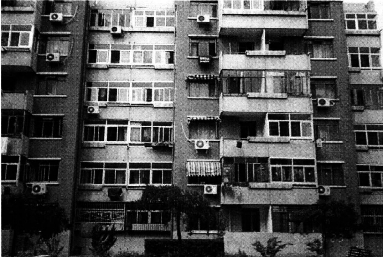
Fig. 7.1 Typical multi-apartment building in Beijing. No insulation, single glazed windows, and poor shading / passive solar design result in high heat losses in winter and overheating in summer.
