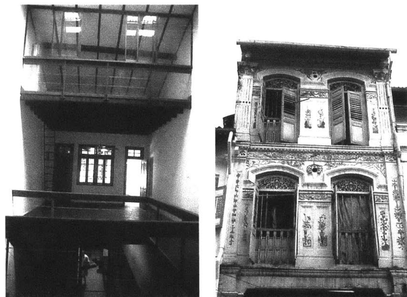
Fig 42 & 43. Interior and exterior façade of typical Shop House
