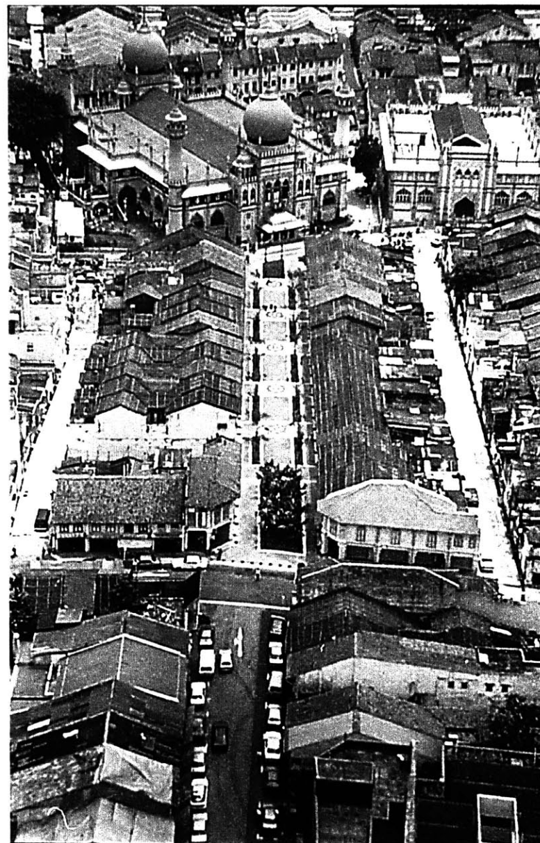
Fig 38. The Bussorah Street Project
