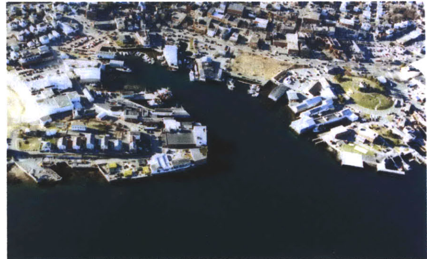
Fig. 6.5 Aerial view of Harbor Cove.
