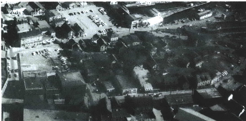
Fig. 3.2 Duncan's Point, now Harbor Loop, prior to Urban Renewal.
