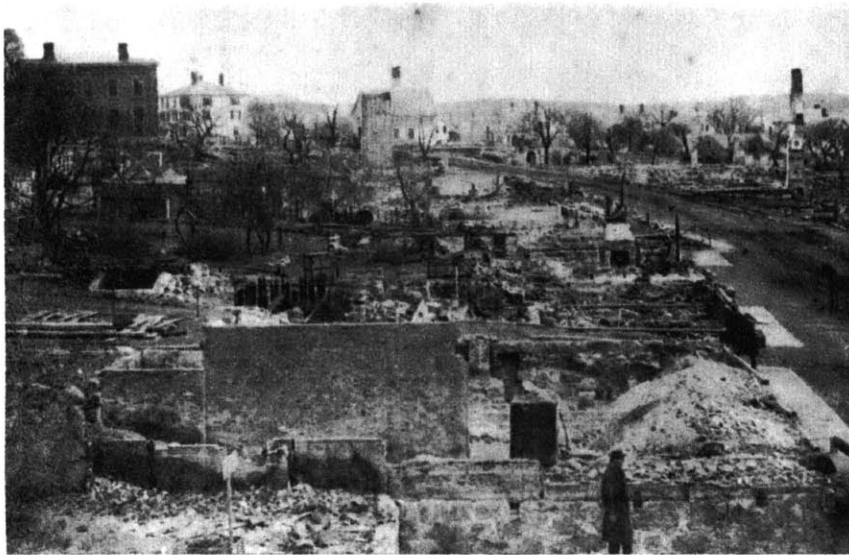
Fig. 2.13 Effects of The Great Fire of February 18, 1864, looking East from the North side of Front (now Main) Street.
