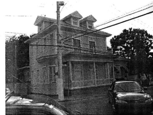
Figure 48: The home of Puerto Rican poet Luis Pales Matos sits vacant along Ashford.
