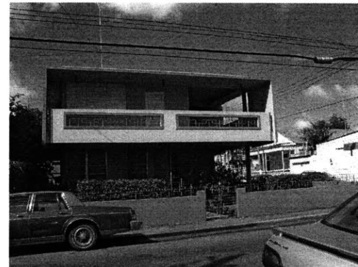
Figure 22: New residential construction before Historic District Designation. Note that the balcony has moved to the second floor and is more private in nature.
