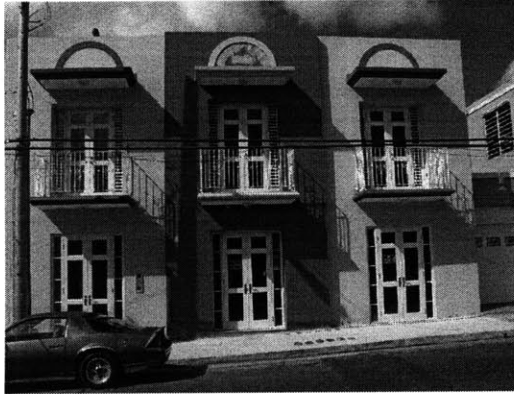
Figure 23: New mixed-use construction using Historic District design guidelines
