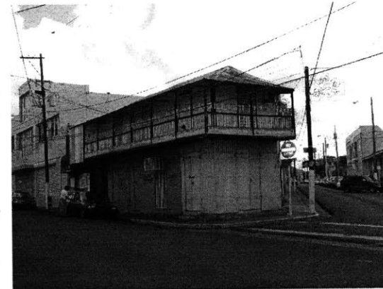
Figure 62: Before - A dilapidated building at a major gateway to the pueblo.
