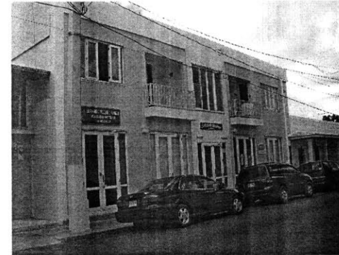
Figure 52: An apartment building along Baldorioty with professional offices on the ground floor.
