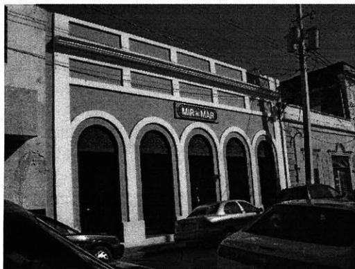
Figure 41: Some locally-owned businesses, have successfully restored their historic commercial buildings.
