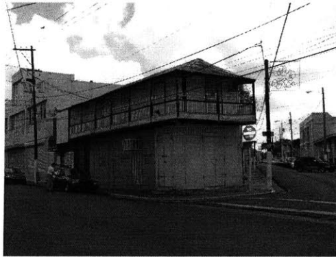
Figure 31: Dilapidated buildings at the entrance to the historic pueblo convey a sense of abandonment to visitors.
