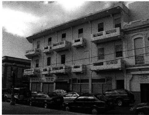
Figure 37: Prominent buildings along the plaza have the potential to support real estate development activities and spur the revitalization process.
