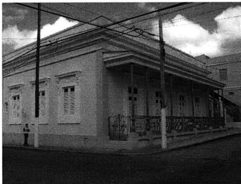
Figure 28: A restored home on the corner of Baldiorioty and Hostos Streets sits vacant.
