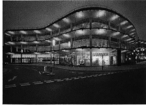
Willis Faber Building, Ipswich, 1975.
