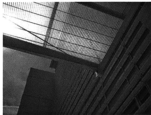
Phoenix Federal Courthouse: Entrance Canopy
