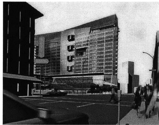
San Francisco Federal Office Building, Morphosis, 2005.
