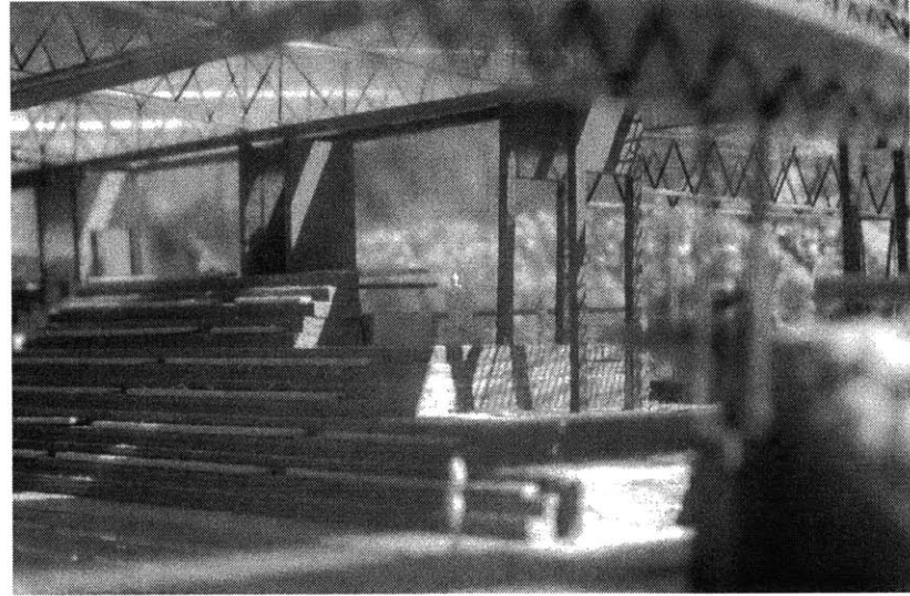
A cafe is located at the end of the spectator stands. Tables in this area have views of the main pool to the north and the recreational pools on the south side.
