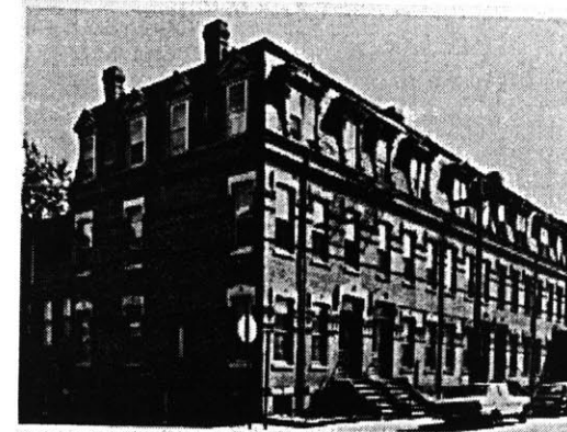
fig.22, row houses at Pearl and Green Sts.
