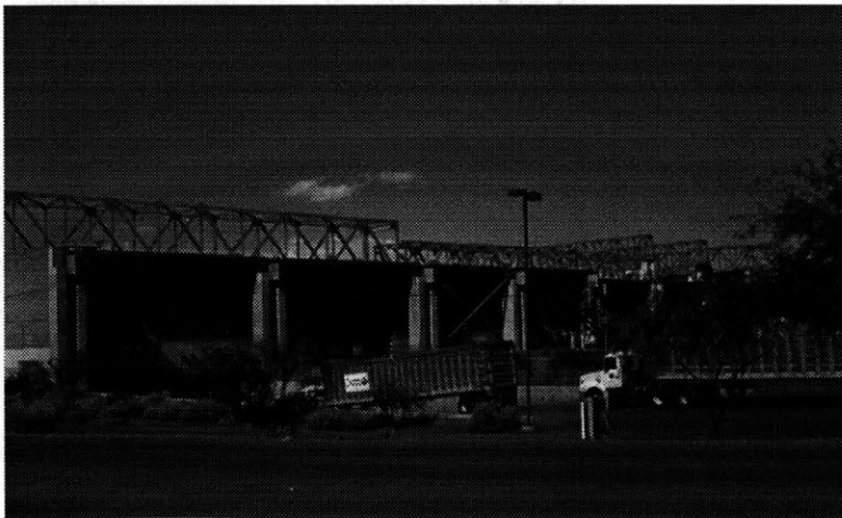
transfer trucks waiting to drive under tipping floor to receive garbage
