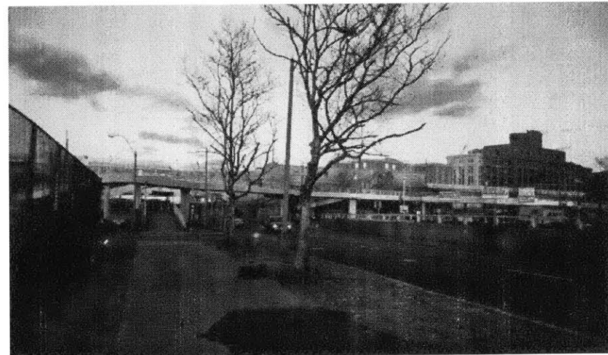
Existing site condition facing southwest
