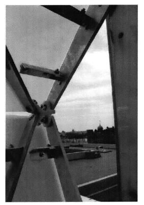
*Figure 084:* Detail at main hinge connection - system closed
