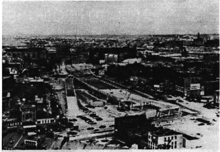
Figure 1.3: Existing Artery Under Construction, 1954.
