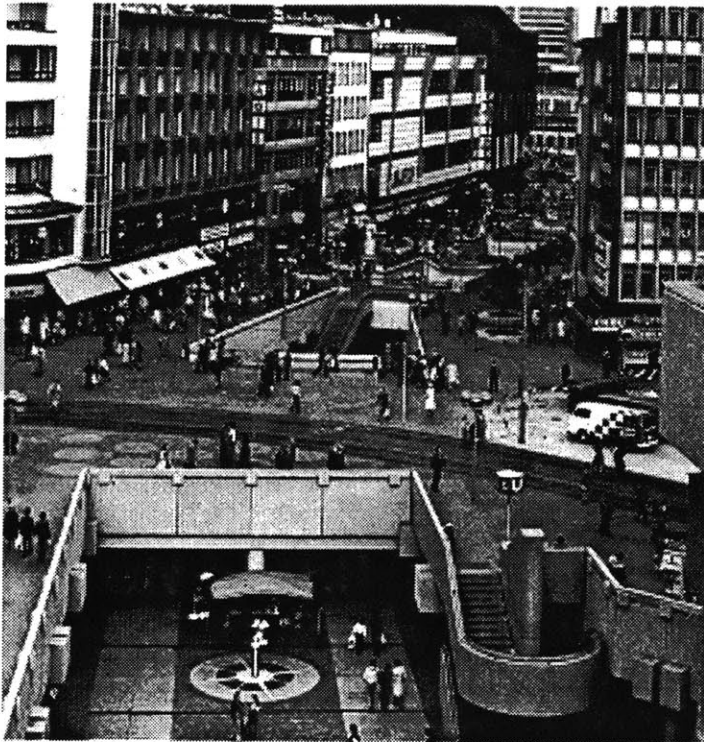
Figure 6.37: Multi-level Pedestrian area in Passerelle, Hanover. [photo from Pedestrian Area, p. 63]
