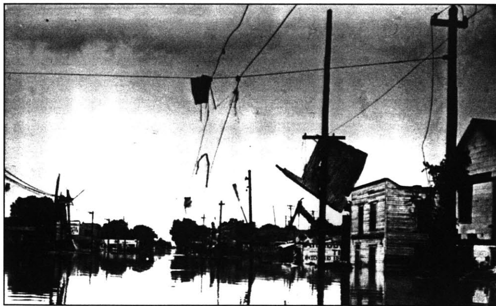
Figure 2.15. Kansas Avenue, Armourdale, View West, early August 1951. Only when the floodwaters finally receded did the full extent of the damage become apparent. Most homes were destroyed, while basic infrastructure and public utilities, including electricity, telephone, electric streetcars, and storm sewers, required substantial repair. (Kansas City, Kansas Police Department Photograph, Kansas State Historical Society, Collection K.2.W7.K.4, #42.)
